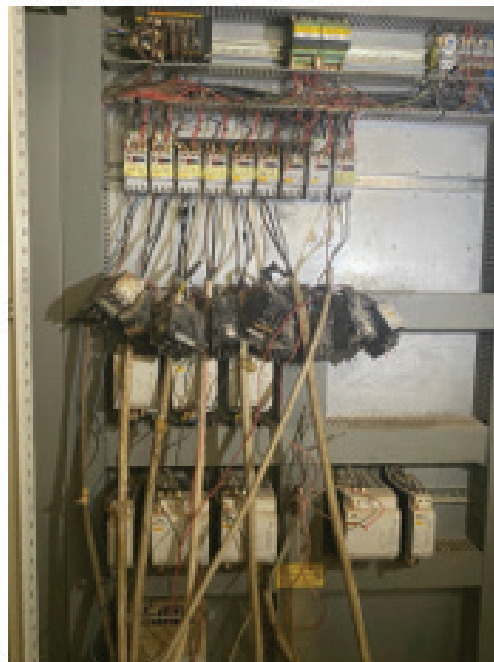
Contractors for the automated aeration system faulty and in state of disuse
