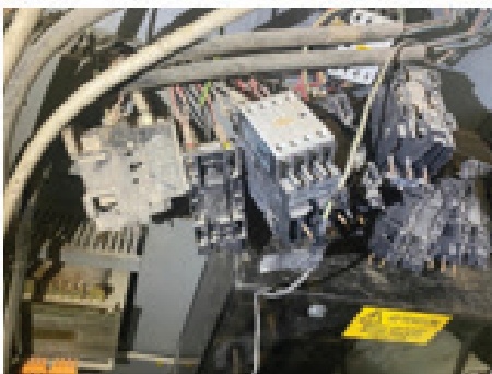
Contractors for the automated aeration system faulty and in state of disuse
