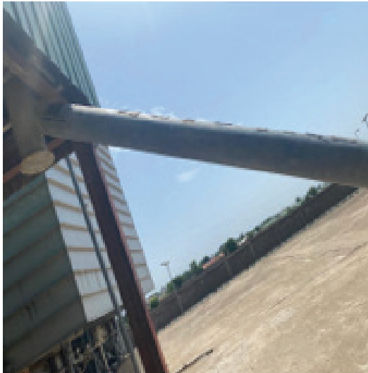
Chute connecting the Cleaner to teh Central Elevator patched so many times to manage its usage
