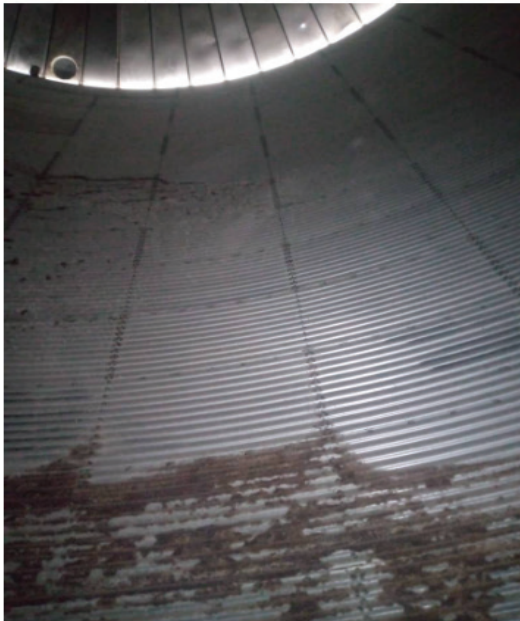
Rusty Inner Wall of the at Irrua Silo
