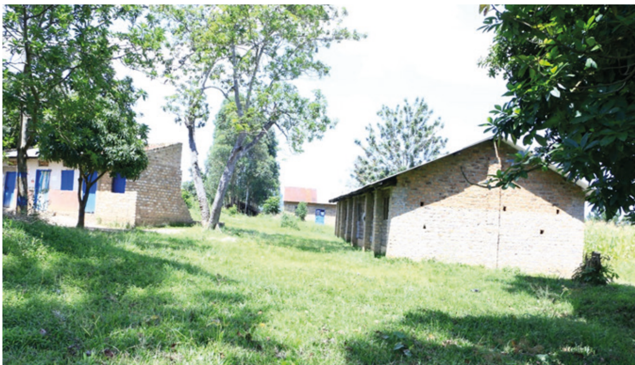
Newly constructed classroom blocks Justine's school, which is about 6 Km from Mubende municipality. Landmark Media Consultancy/Joseph Buule.
